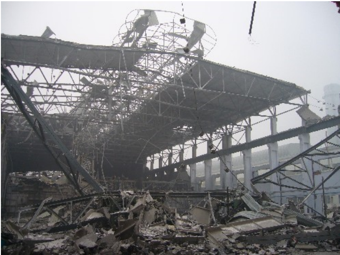
Figure 5. August 19, 2007, Explosion occurred when furnace lining failed and contents emptied into casting pit.
