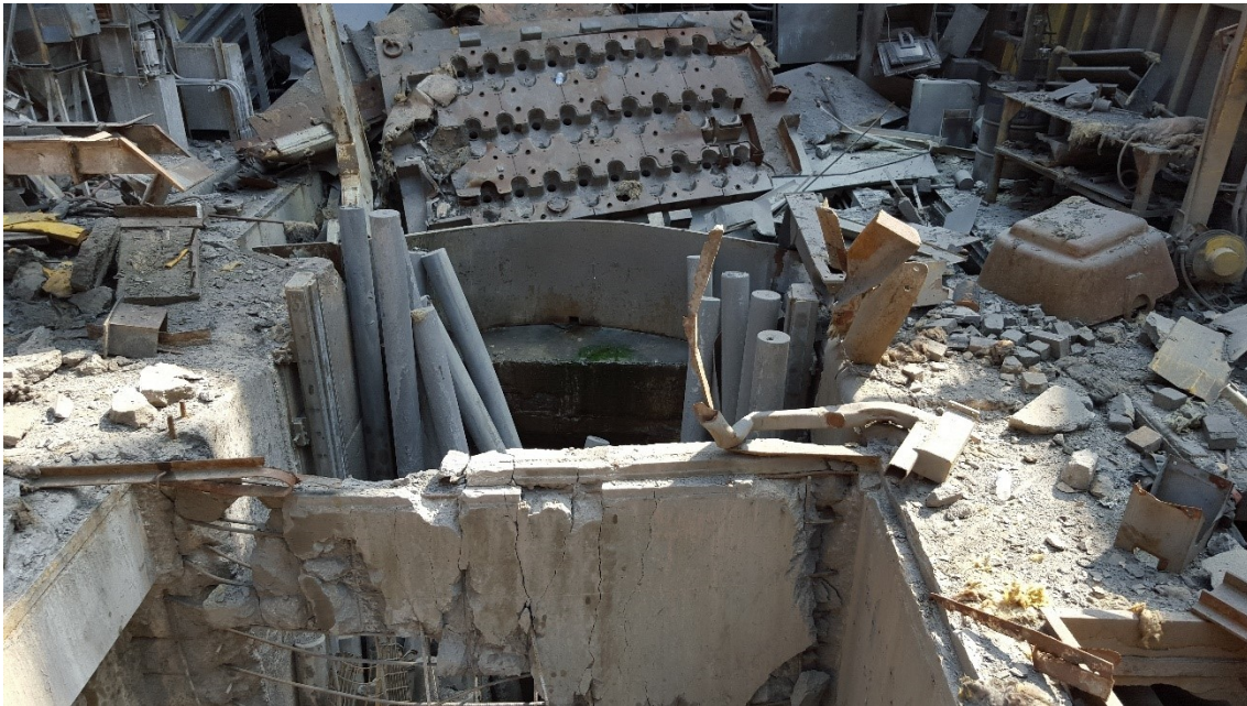
Figure 6. August 4, 2015, Noranda Aluminum explosion.
